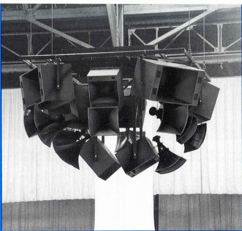
View of Main Loudspeaker Array
